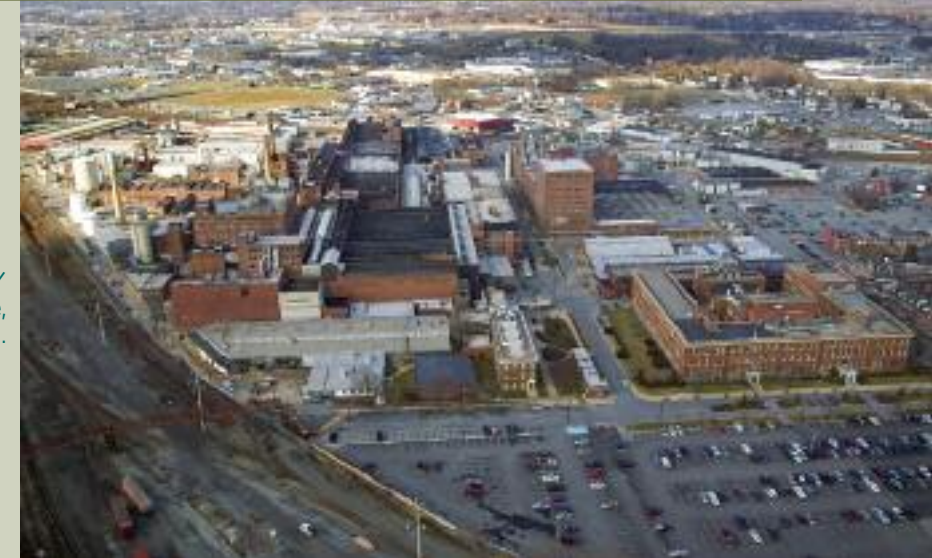
Northwest Gateway Project/ Armstrong World Industries site, shown in February 2005...
